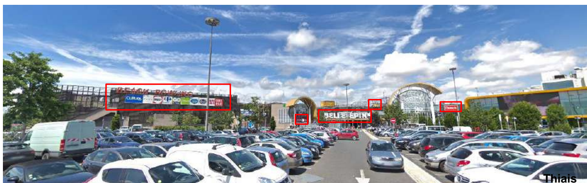
Centre commercial Belle Epine – Thiais – Source : Google Streetview
